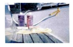
4. You now have 2 alternatives. If you do not have aluminium in the area you can rinse away liquid No.1, with water. Before rinsing however, wait a few minutes so that SNAPPY can work deep down in the wood. If, however, you do have aluminium use alternative number 2. which is to apply liquid No.2. directly on top of liquid No1 without rinsing. This creates a neutral mixture which cannot effect aluminium when it is rinsed off at a later time. This mixture is also better for the environment.
