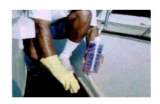
3. Apply No. 1, using brush No. 1. Brush across the grain using a force equal to that force you use when you wash your hands. Do not mix the brushes as the two liquids(No.1&2) neutralize each other. If SNAPPY begins to dry into the deck (sunny day) spray lightly with water. SNAPPY works only in a wet environment. Do not be afraid that your deck turns almost black in color. That indicates SNAPPY is working.
