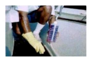
5. The next step is to apply liquid No.2. Use exactly the same technique as used when applying liquid No.1. Almost immediately your deck will begin to lighten in color. Again wait a few minutes so the liquid can work deep down.
